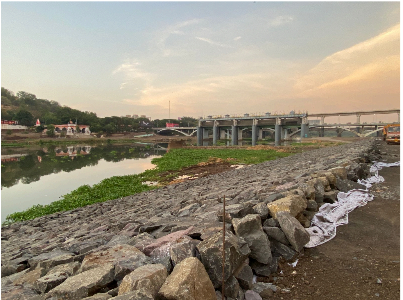
Creation of artificial banks by laying rocks along the banks of the Mula Mutha (Image Source: Jeevitnadi)
